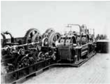
CABLE LAYING MACHINERY: It was as a cable layer that the Great Eastern finally found her calling.
