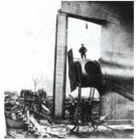
PROPULSION: The sternpost screw on the Great Eastern was large but not enough to propel the giant ship, so Brunel had to revert to paddlewheels and sails in addition.
